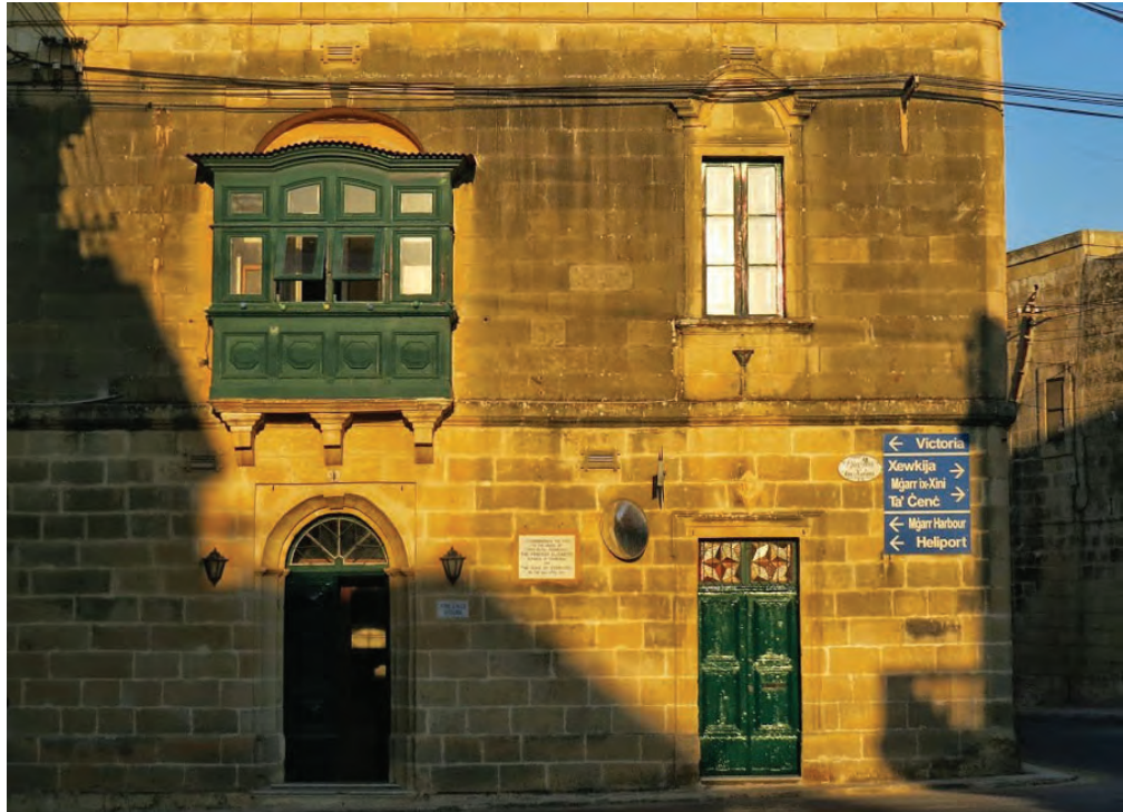
Figure 85: Openings located on buildings within older village cores are typically characterised by symmetrically positioned vertical openings organised in horizontal bands and a high solid: void ratio
