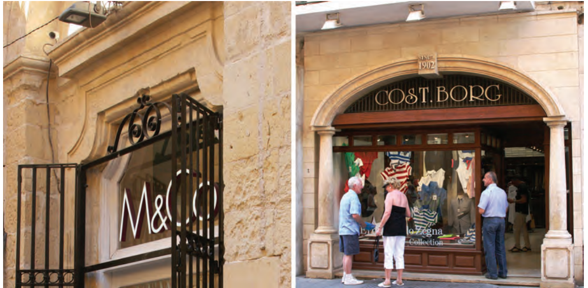
Figure 77: Well-designed shop front illumination
