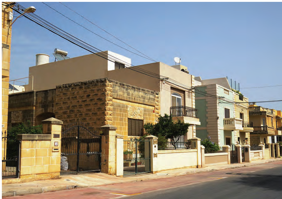
Figure 27: Well-proportioned front garden boundary walls
