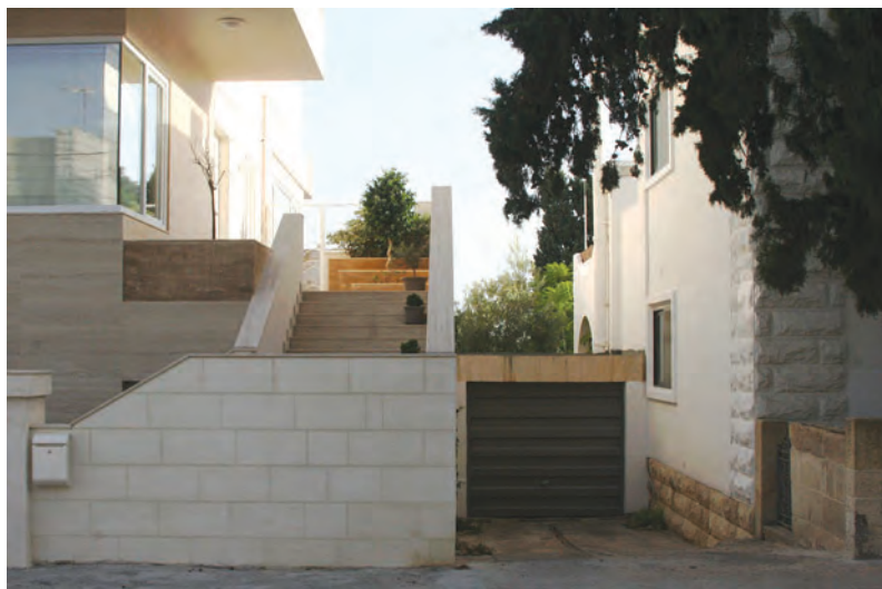
Figure 36: Garage within the side curtilage
