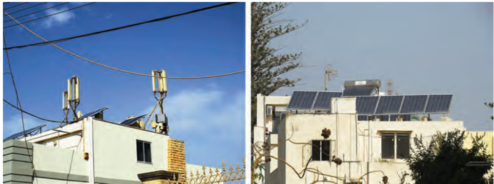
Figure 93: Visual clutter on roofscapes due to the sporadic location of services
