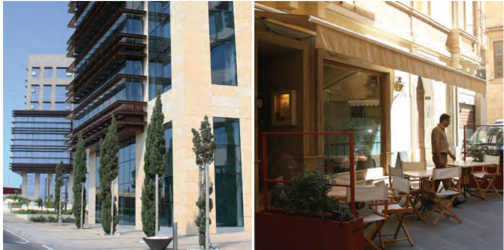
Figure 74: Canopy/shading device (left) and retractable awning (right) deployed on the façade of buildings
